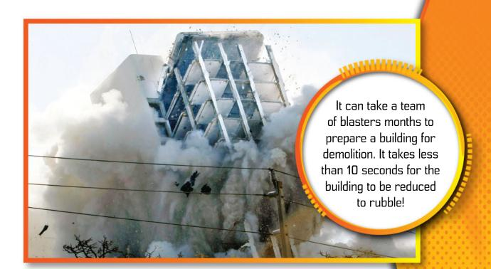
Blasters are highly skilled **engineers** who rig a building with **dynamite**. The explosive **charges** are placed with absolute precision to ensure that a building collapses within a specific area. When the explosives are **detonated**, the building's framework must shatter. Then **gravity** does the rest!
