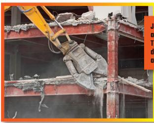
Jaw-like tools are attached to an excavator's boom, or arm. These powerful tools can tear down walls, crush concrete, and cut through steel.
